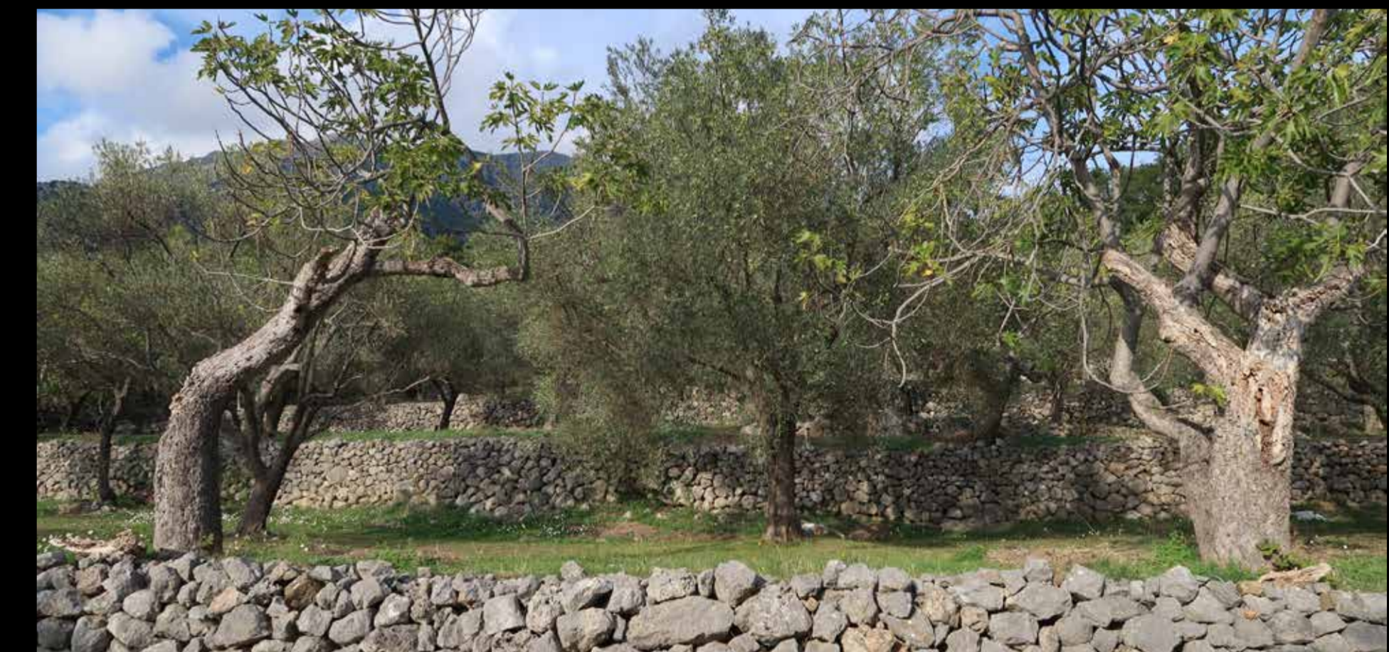
2 - Dry-stone walls of terraced dales with olive groves, Dobro vode, Bar
